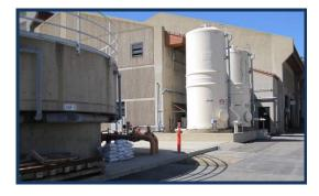
The Emulsion Polymer Upgrade Project was part of the Regional Treatment Plant Miscellaneous Improvements 2011 Project. Existing polymer pumps and piping were relocated inside the existing building. Challenges included sequencing construction to maintain plant operation.
